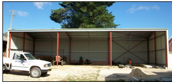
...and the new farm and machinery shed.
