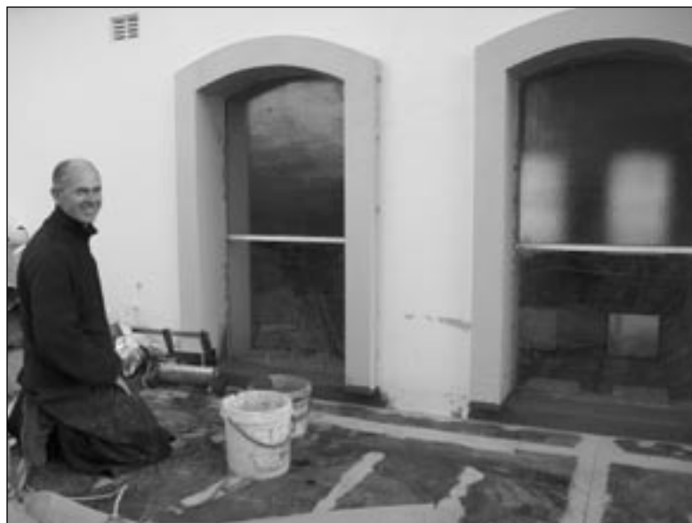
Brother Joseph works on the roof adjacent to the chapel
