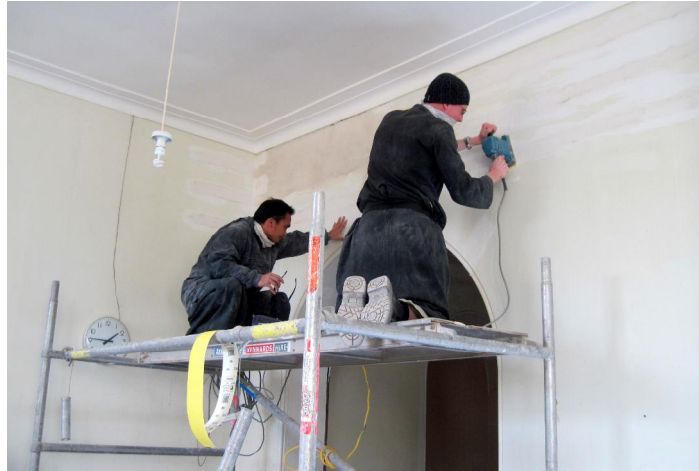
Sanding the scars left by the repairs
