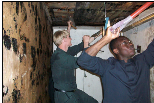
Gutting the walk-in Refrigerators
