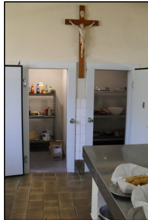
The newly refurbished Refrigerators
